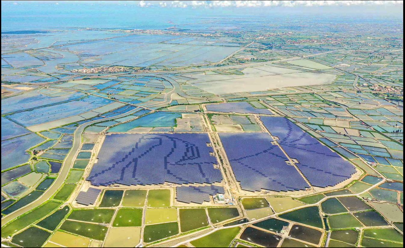
Vena Energy's 70 MW Mingus Solar Project
